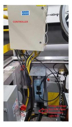
Technicians must switch off the circuit breaker in the Foreign Voltage Box (Upper Demarcation Light Box) shown below.
