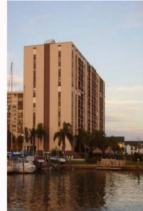
Dolphin Cove Condominium
